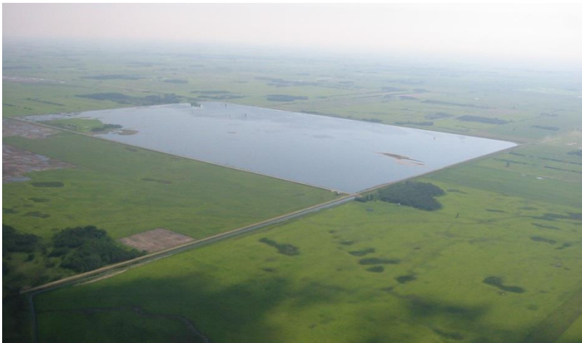
Typical Water Retention Site During Spring Operation
